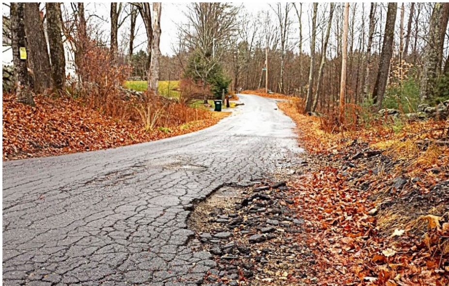
Photo 2: Edge Cracking on Thornton Rd (photo credit: Anthony Summers)
