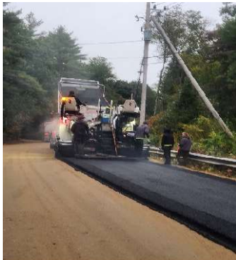
Paving of Reclaimed Twin Bridge Road
