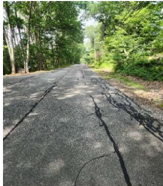
Crack Sealing on Old Coach Road
